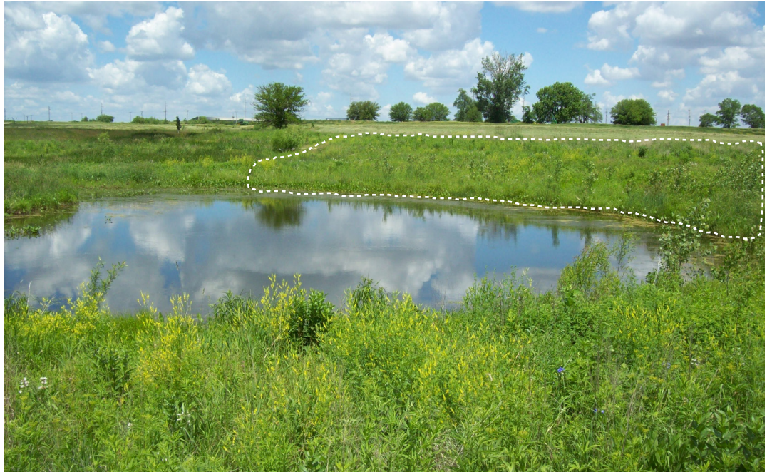
Filter strip around a constructed stormwater wetland.
