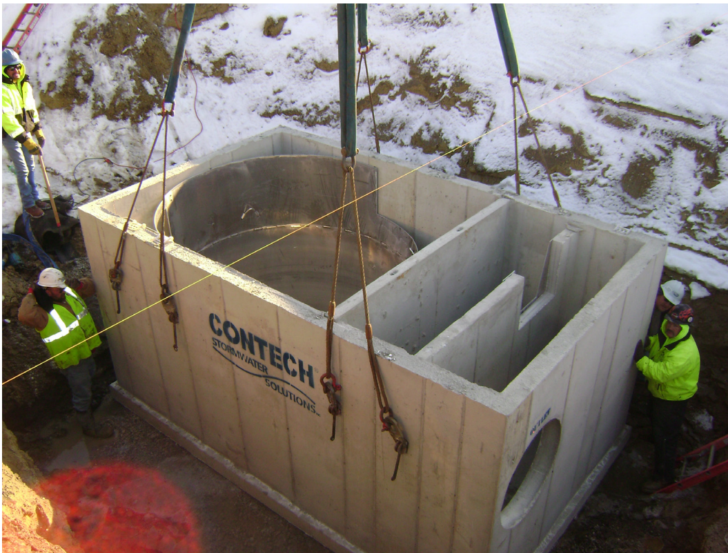
Installation of a hydrodynamic separator.
